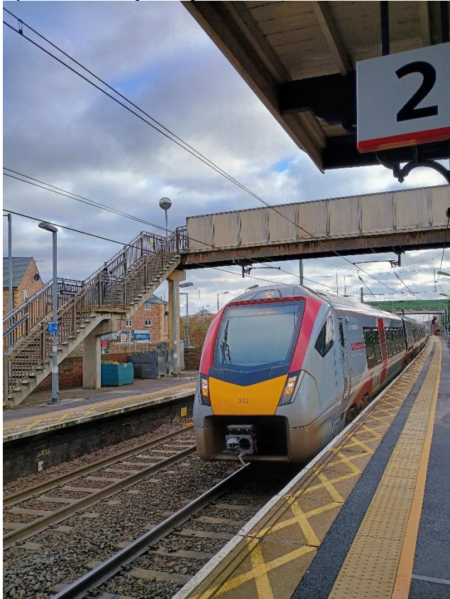
The old footbridge at Stowmarket
