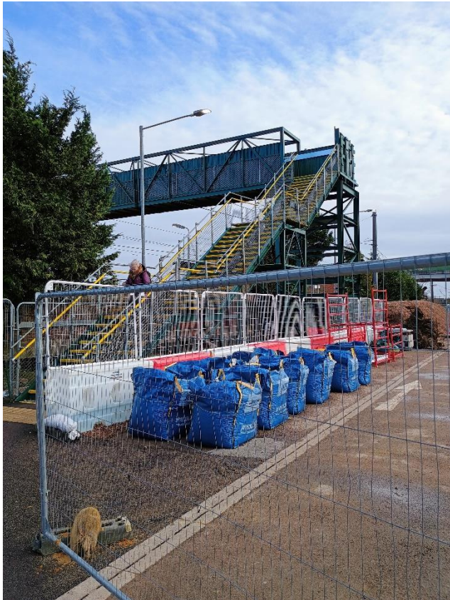
The worksite compound
