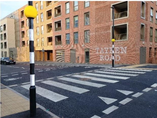
The new Tayfen Road pedestrian crossing.
